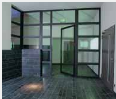
T30 door, single leaf, with lateral part and top light
