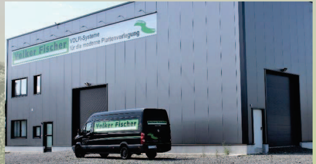
Plant 3 VOLFI logistics centre
