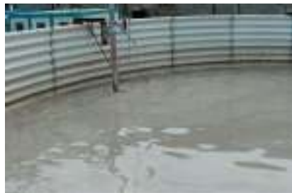
Processed drilling fluid
