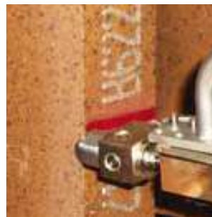
Chimney stone line-marking for correct installation
