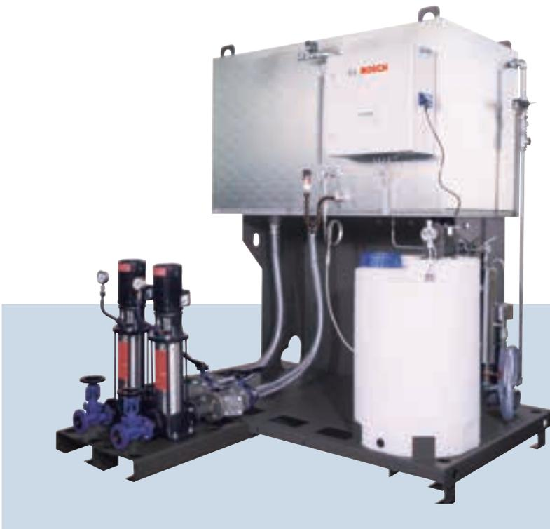
Water service module WSM-T for partial deaeration for all steam boilers with capacities of up to 8000 kg/h
