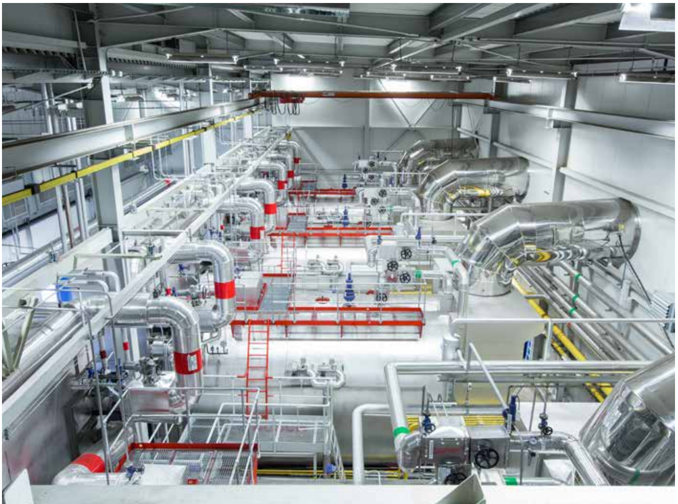
The four ZFR-X steam boilers each have an operating weight of 145 tons.
