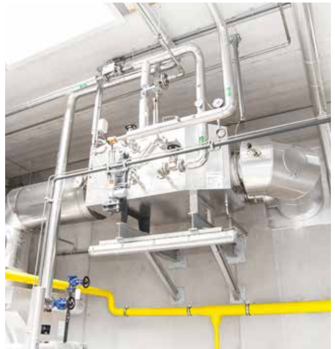
Flue gas heat exchanger ECO 6 for condensing use
