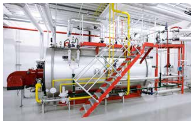
The new, modular steam boiler UL-S with heat recovery equipment for maximum efficiency.
